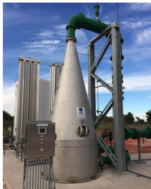
Figure 6 - ECO 2 's Application of the Speece Cone (ECO 2 Oxygen Technologies, 2020)
